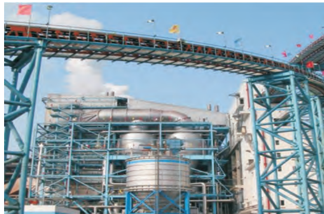
电站锅炉管 Utility boiler tube
