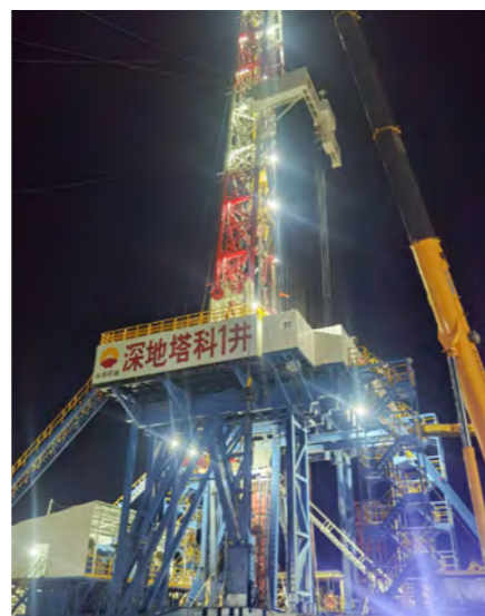
Casing steel from Baosteel was successfully deployed in Shenditake 1 at CNPC's Tarim Oilfield, supporting successful downhole installation at extreme depths.
