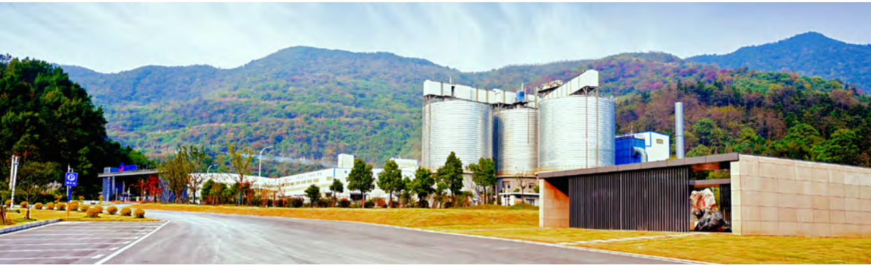
宝武资源安徽皖宝投入 927.77 万元，实施桃冲青阳矿环境整治、秀山矿绿色矿山建设，矿区环境大幅改善。 Baowu Resources' Anhui Wanbao invested RMB 9.2777 million for the environmental renovation at the Taoshong Qingyang mine and the green mining construction at Xiushan mine, significantly improving the mining environment.
