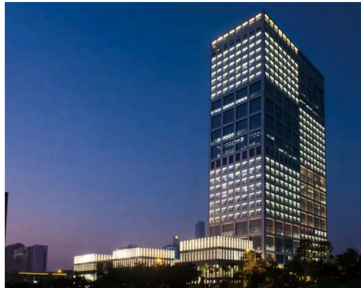
中国宝武广州宝地广场获评全国首批零碳数智楼宇试点单位。 China Baowu's Baodi Plaza in Guangzhou has been recognized as one of the first batch of zero-carbon smart building pilot units across the nation.
