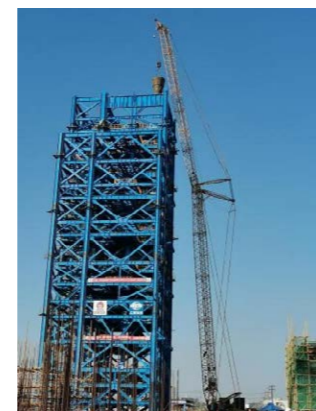
The first hoist of shaft furnace shell
