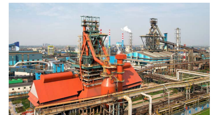
No.1 Furnace Picture of Wugang
