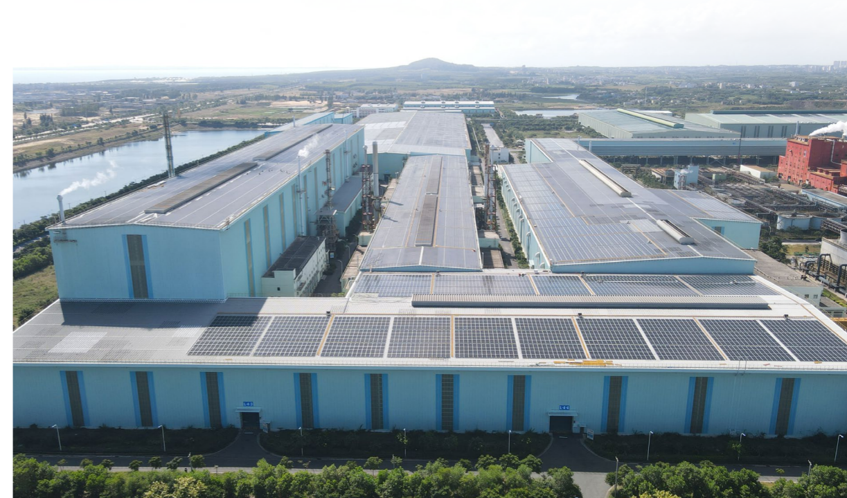
宝钢股份湛江钢铁屋顶光伏项目 Rooftop Photovoltaic Project of Zhanjiang Iron and Steel of Baosteel
