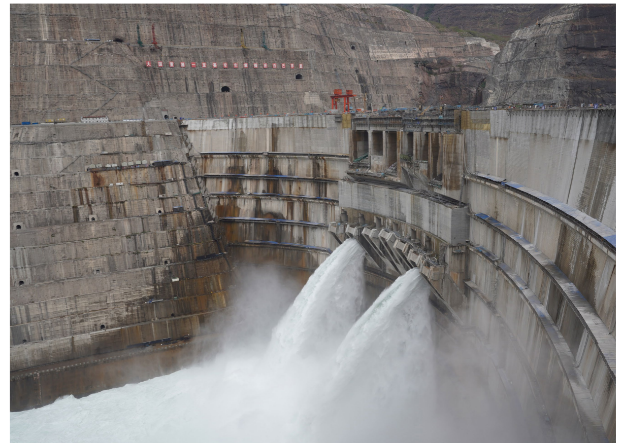
● “国之重器”白鹤滩水电站 "National Pillar" Baihetan Hydropower Station
